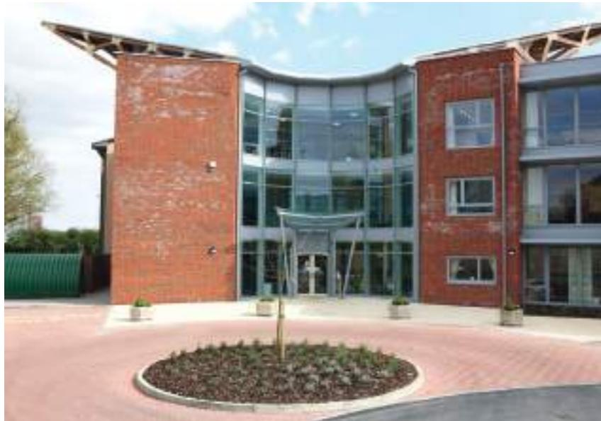
To help realise their ambitious plans, the main contractors, Baxter & King Construction, specified an internally faceted three-storey screen using the REHAU Polytec 50 composite curtain walling system.
